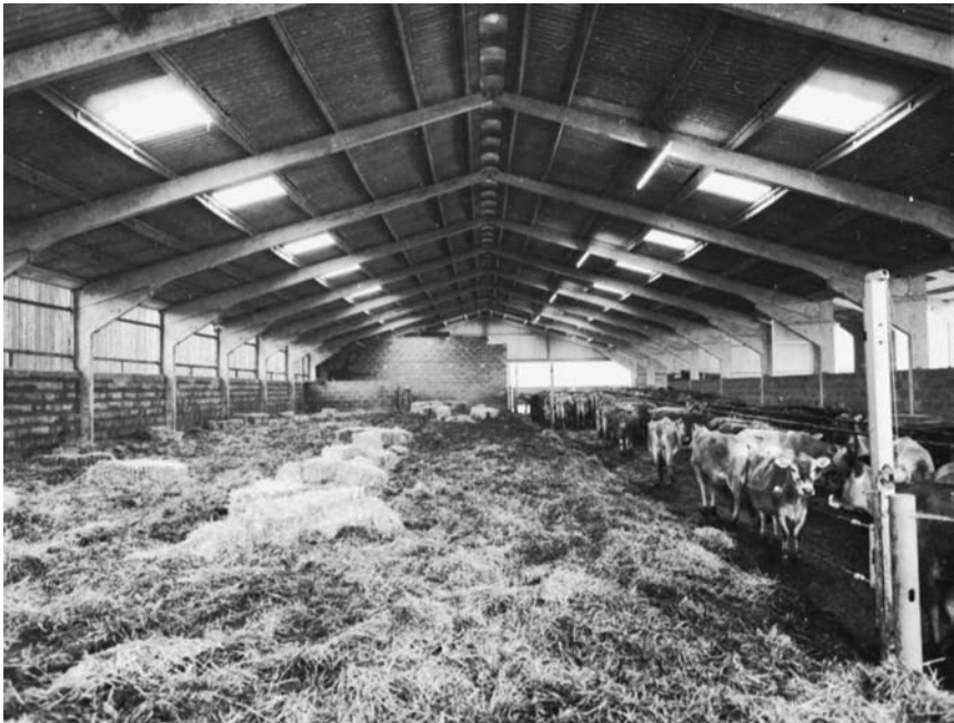
A dairy unit, with lying area, parlour and dairy under one roof. Note the Yorkshire boarding to the left of the picture — a means of ensuring good ventilation and an absence of condensation.
